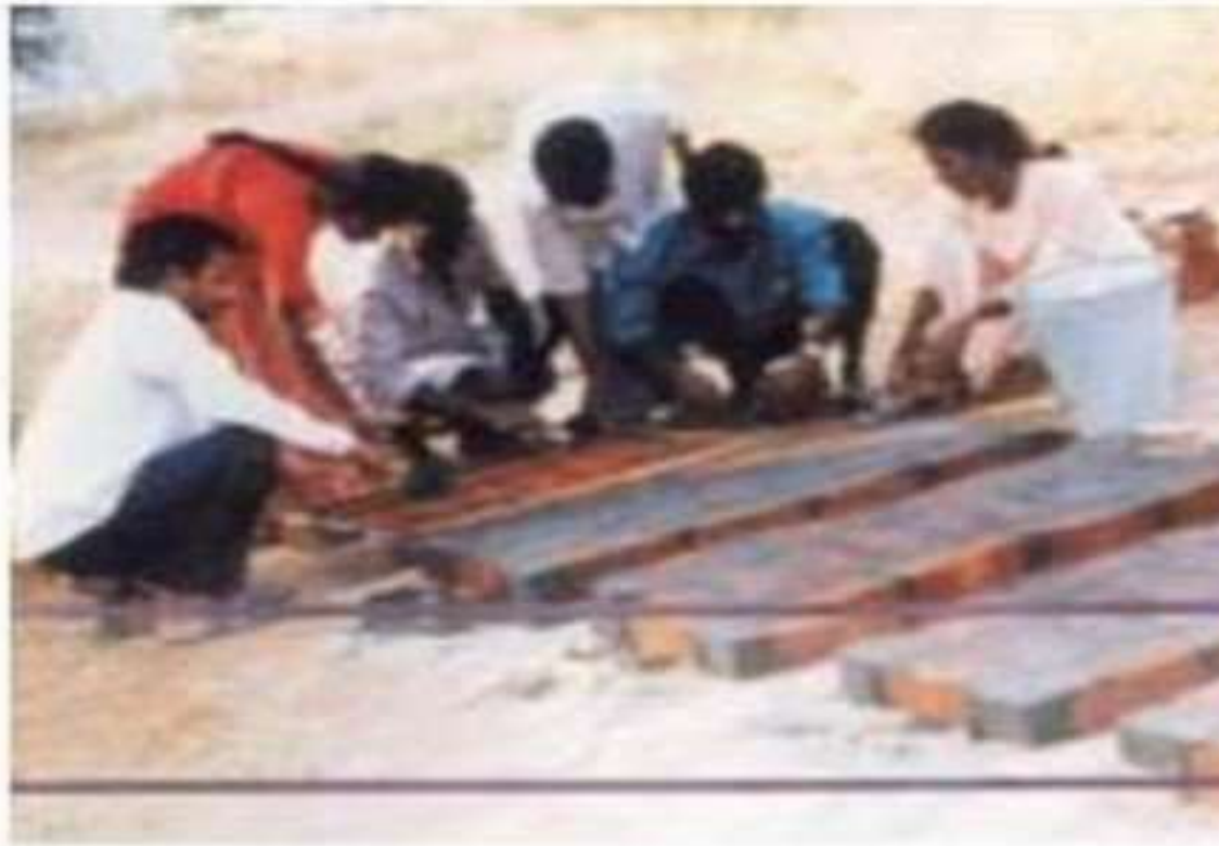
Image 2: Prefab brick panels. (picture taken from [unclear])
